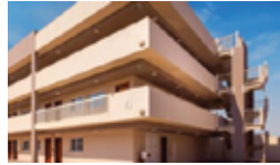
Khalifa City & Al Sader Rapid Intervention Bld., Abu Dhabi
