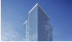
Al Huwailah Towers at Al Mirqab, Qatar
