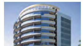
Commercial & Residential Building at Al Qusais Ind, Dubai
