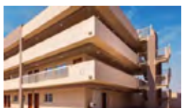
Khalifa City & Al Sader Rapid Intervention Bld., Abu Dhabi
