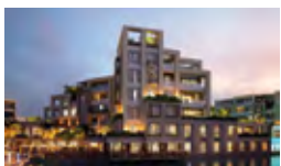
Deira Water Front Development, Dubai
