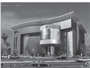
Dubai Municipality Offices Dubai - U.A.E.
